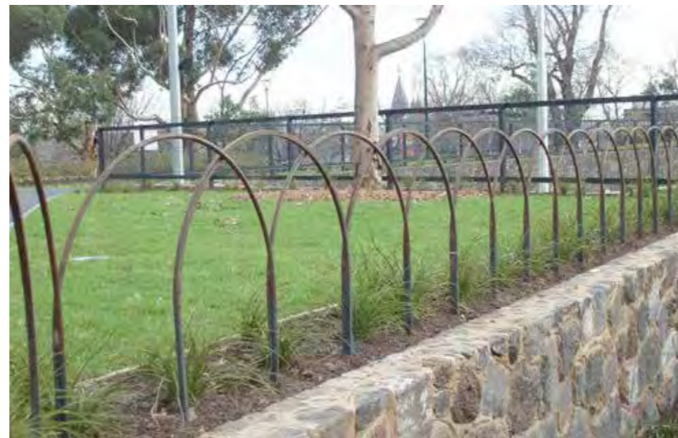
TEMPORARY FENCING: MILD STEEL HOOP FENCING
