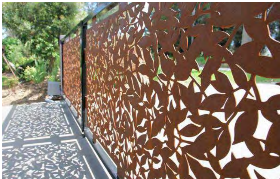
02 - THE TIN ALLEY ACCESS WILL HAVE A NEW SLIDING GATE, MADE FROM LASER CUT CORTEN STEEL
