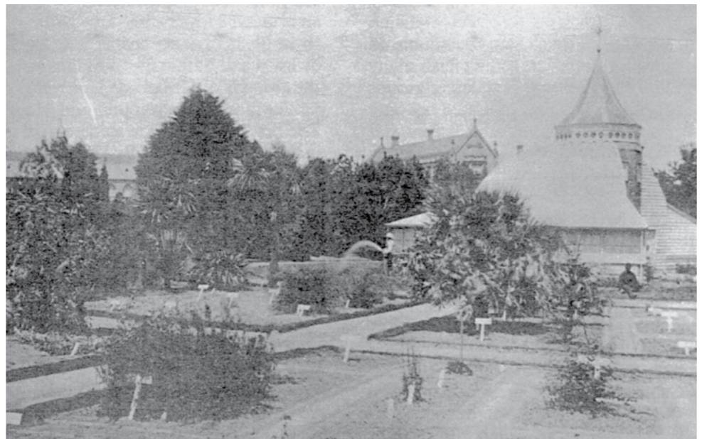
1873 PHOTOGRAPH OF THE SYSTEM GARDEN AFTER THE INSTALLATION OF THE GLASSHOUSE, PHOTOGRAPH BY G NETTLETON. SOURCE: G PASCOE/UOM ARCHIVES
